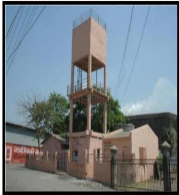
Overhead water tank of Baben
