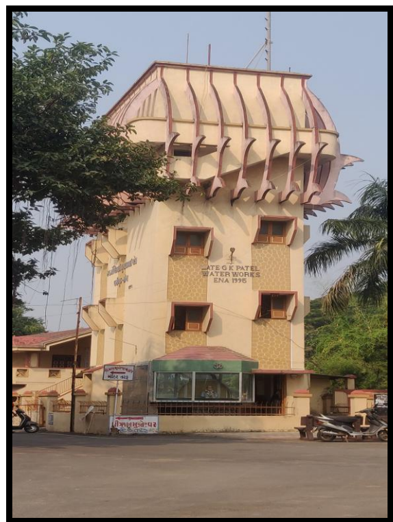
Overhead water tank of Ena
